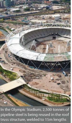
pipeline steel is being reused in the roof truss structure, welded to 15m lengths from 12m stock. (Image: London 2012)
