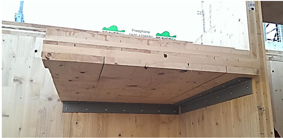
Fig. 16 Special moment connection for a cantilever stair half landing slab.
