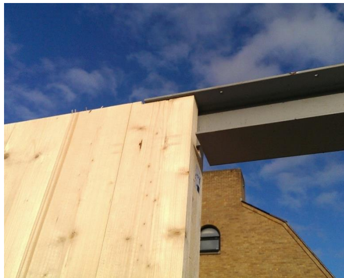
Fig. 17 Special detail to support end bearing of a steel lintel beam.
